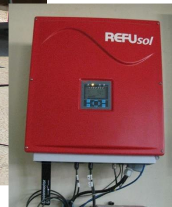
PV Inverter (REFUsoI 010K)
