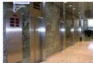
Turn off 1 of 4 elevators
