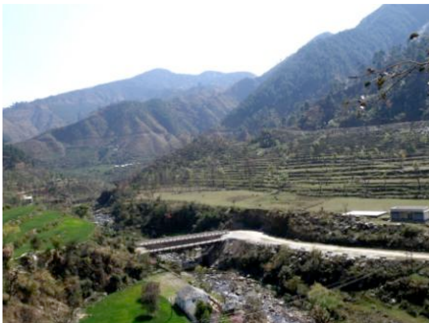
The bridge to IIT Mandi
